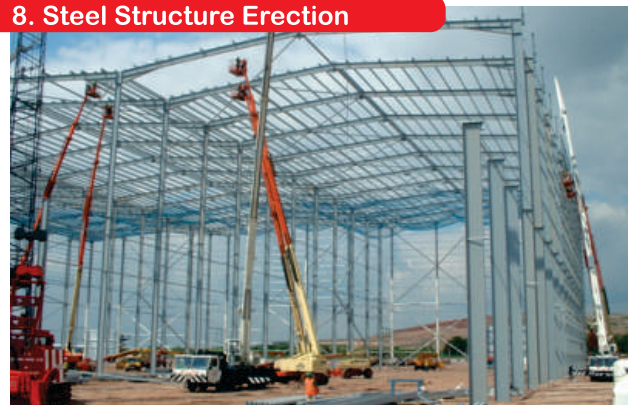
8. Steel Structure Erection
